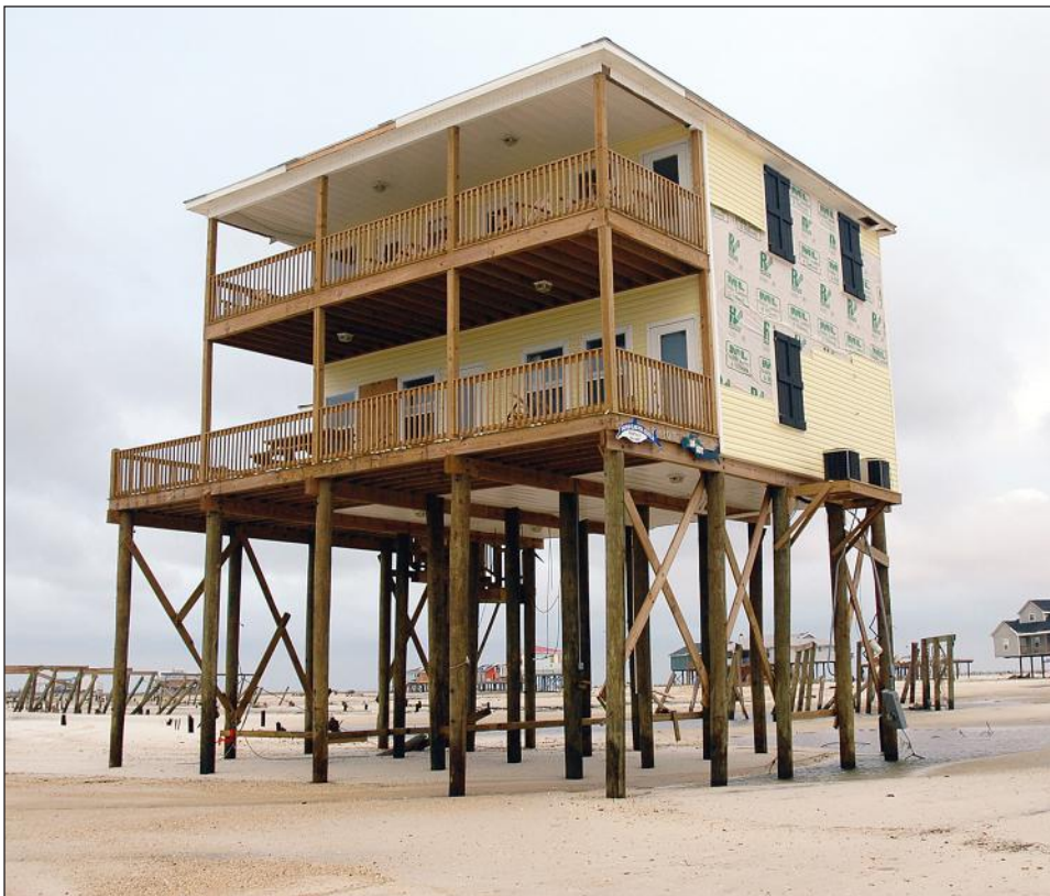
Figure 3-10. Home elevated on piles.
