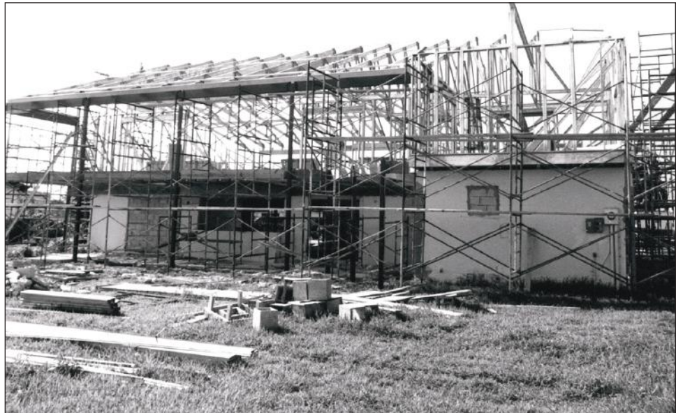
Figure 3-12. The owner of this flood-prone home in south Florida decided to build a new wood-framed second story on top of the masonry first story. The new second story is well above the BFE.
