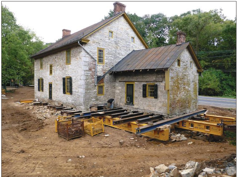
Figure 6-4. Beams supported by cribbing are placed at critical lift points (photo courtesy of Wolfe House Movers).
