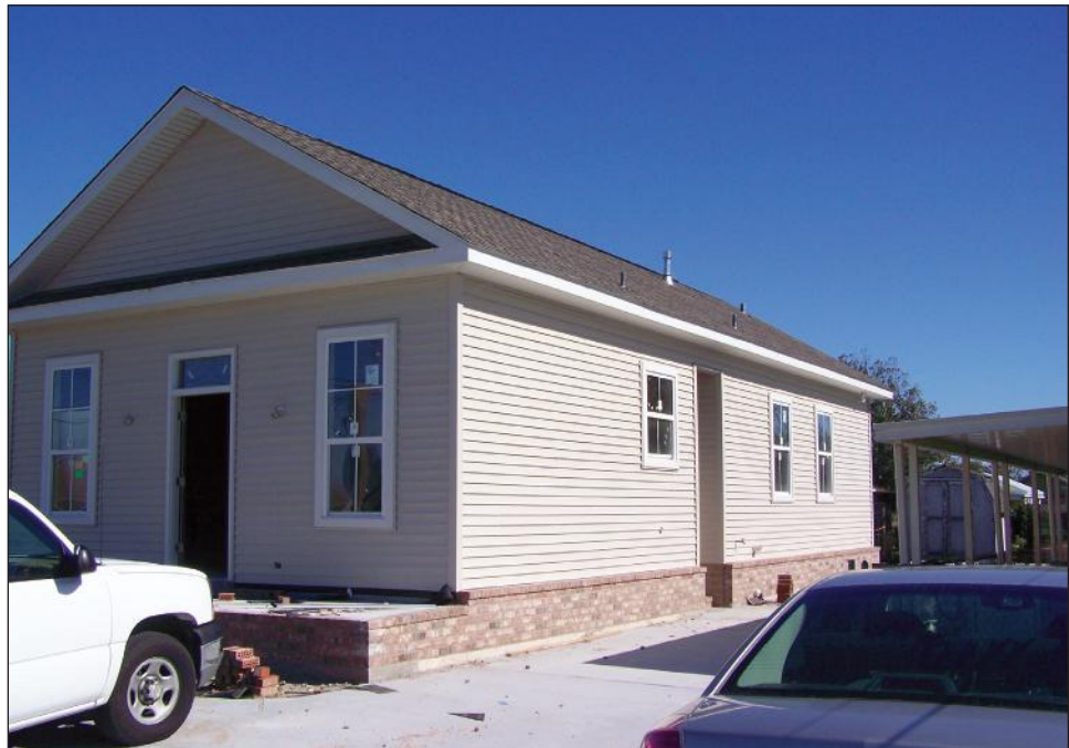
Figure 6-9. Typical mitigation reconstruction project.
