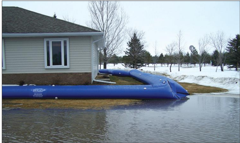
Figure 8-4. Two-foot-high water-filled temporary barrier protecting a residence from flooding (2010 – Courtesy of Hydrological Solutions, Inc.).
