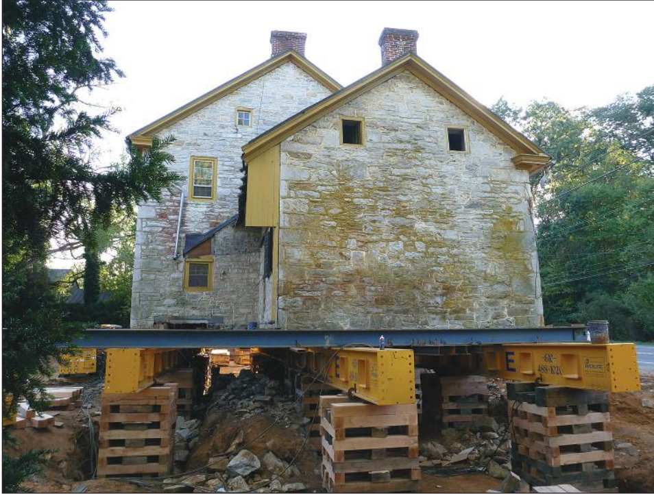
Figure 6-5. Hydraulic jacks lift the structure, and the home is separated from existing foundation (photo courtesy of Wolfe House Movers).
