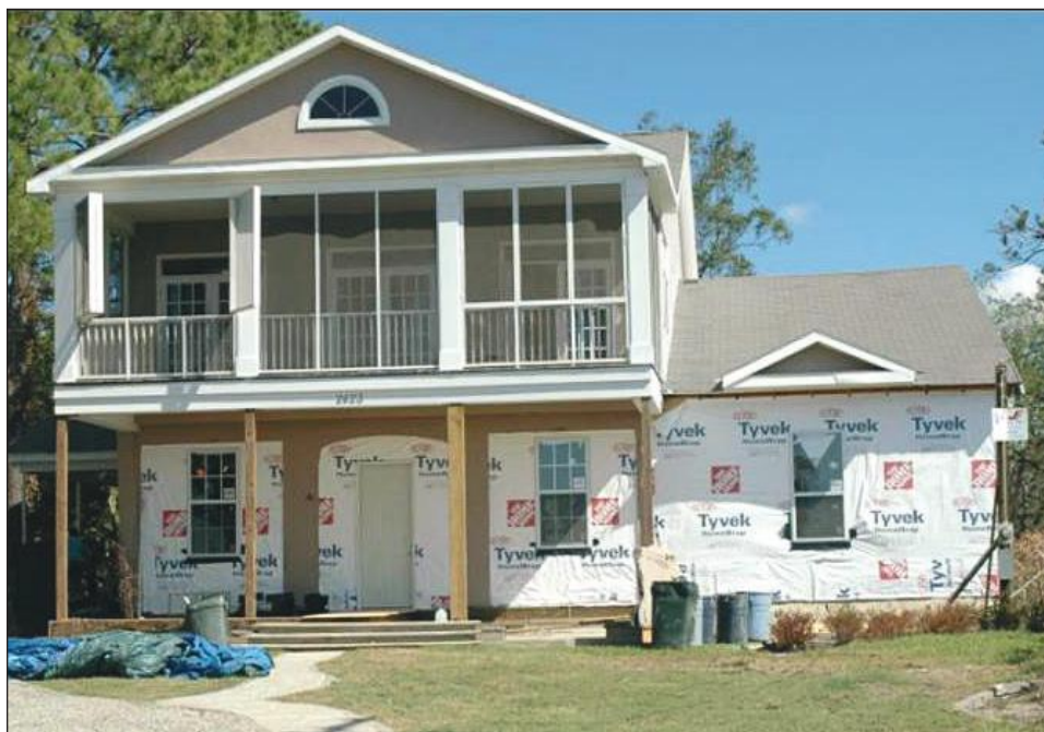
Figure 2-1. This home in New Orleans was inundated by 4 feet of water during Hurricane Katrina.
