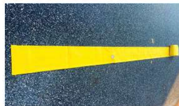
Unroll flood tube sections before filling with water
