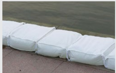
Place First Row of Bags Down, With the Long Side Parallel to Water
