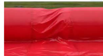
Attaching the Tube Connector Sheets (To prevent leakage)
