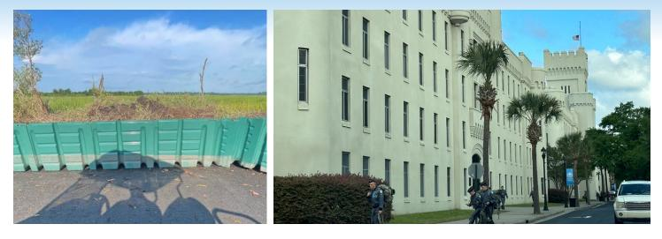
The college acquired both Straight Mayim<sup>™</sup> MB2-S Panels and Curved Mayim<sup>™</sup> MB2-OC Panels, allowing the system to be shaped to follow the corner turns in the parking lots, providing additional protection against water migrating around the panels during higher tide situations.
