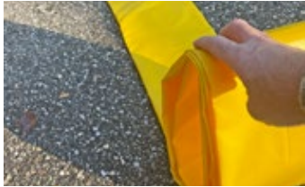
Unroll Guppy Flood Tubes before filling.
