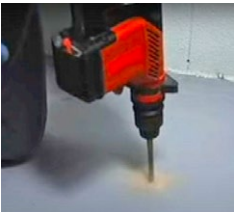
Drilling For Mounting
