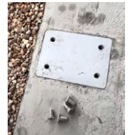
Installed Base Plate
