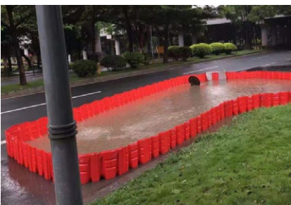
Sewer & Drain Overflow Containment
