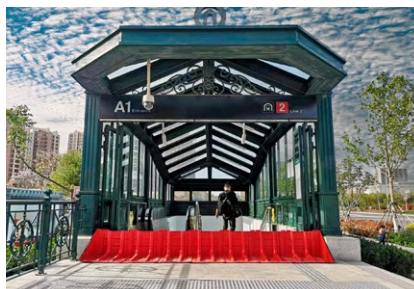
Transit Flood Diversion Barrier
