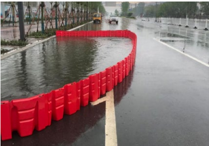
Street Flooding Diversion Barrier
